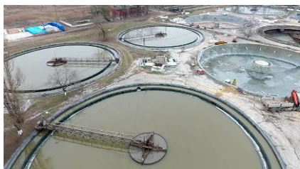
Fig. 7. Chișinău wastewater treatment plant - decanters
