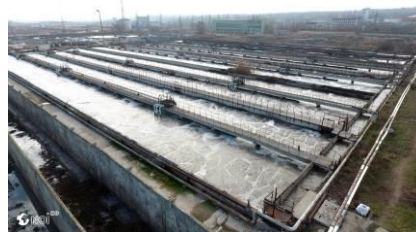
Fig. 8. Chișinău wastewater treatment plant - filters
