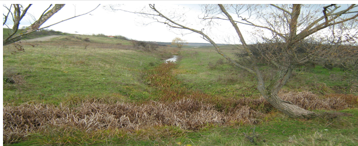
Fig. 3 Infection with vegetation of natural outlets from the perimeters of improvement
