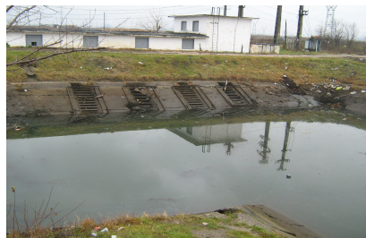
Figure 2: The degraded suction basin of the station
