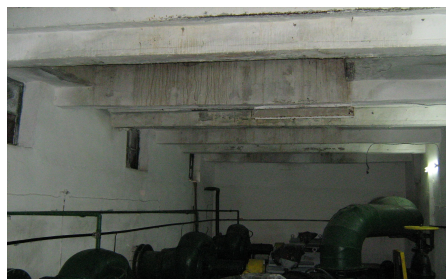
Figure 1: The interior of pumping station, infiltrations and aggregates state
