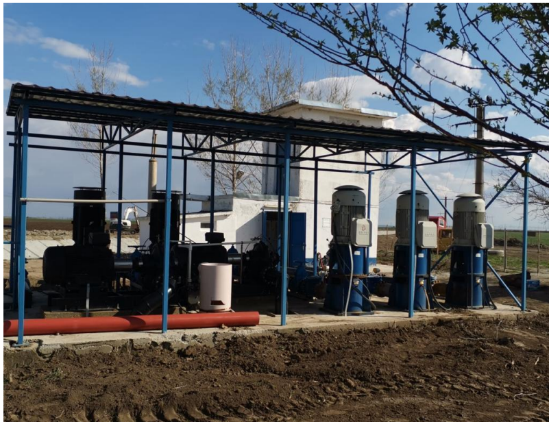
Fig. 7 Side view of new SPP13 electric pumps and pumping station superstructure
