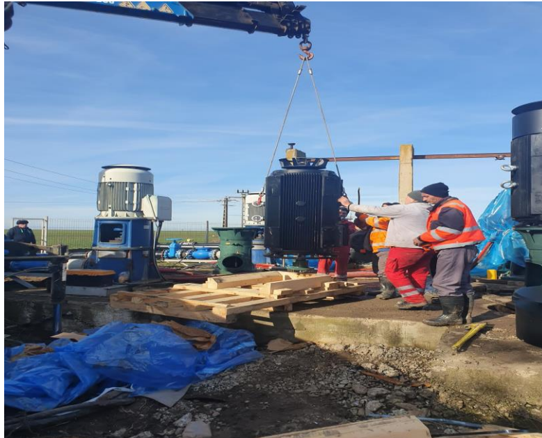
Fig. 6 Detail view - pump transport for position mounting at SPP 13
