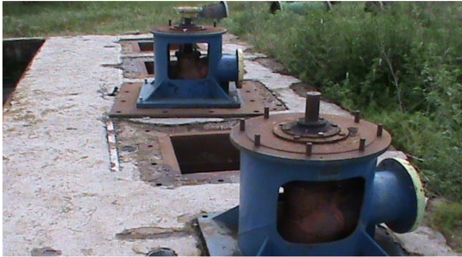
Fig. 2 Detail of SPP 13 pumps disabled
